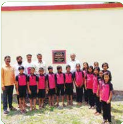
Constructed Ladies and Gents Toilet Block at Innovative School Ankoli Taluka Mohol Dist. Solapur Dt 03.09.2022
